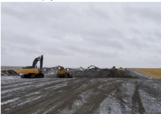
Excavators pulling transition - SF 65 – Nov 5, 2018
