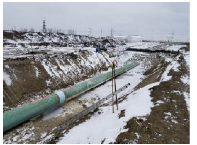
Test and tie-in site – SF 34 – Nov 7, 2018
