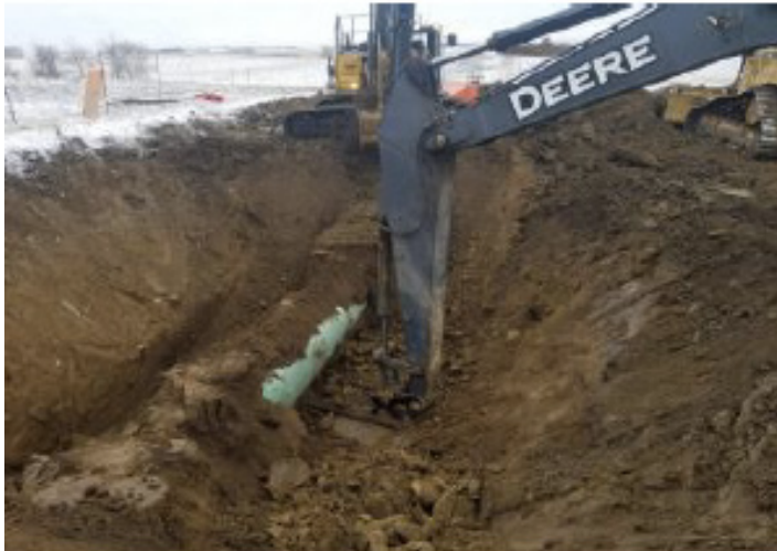
Excavator cleaning soil under pipe - SF 22 – Nov 10, 2018
