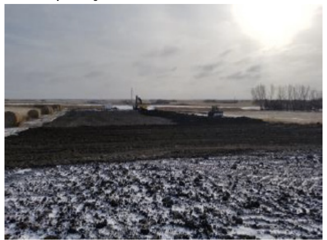
Ovality dig completed– SF 49 – Nov 5, 2018
