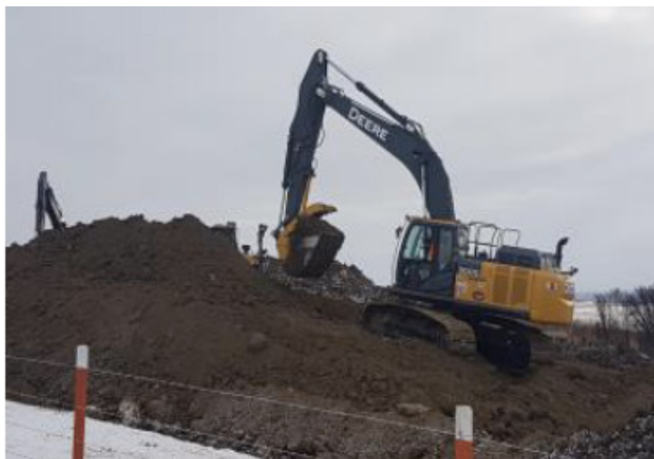
Excavator working on ovality dig - SF 22 – Nov 8, 2018
