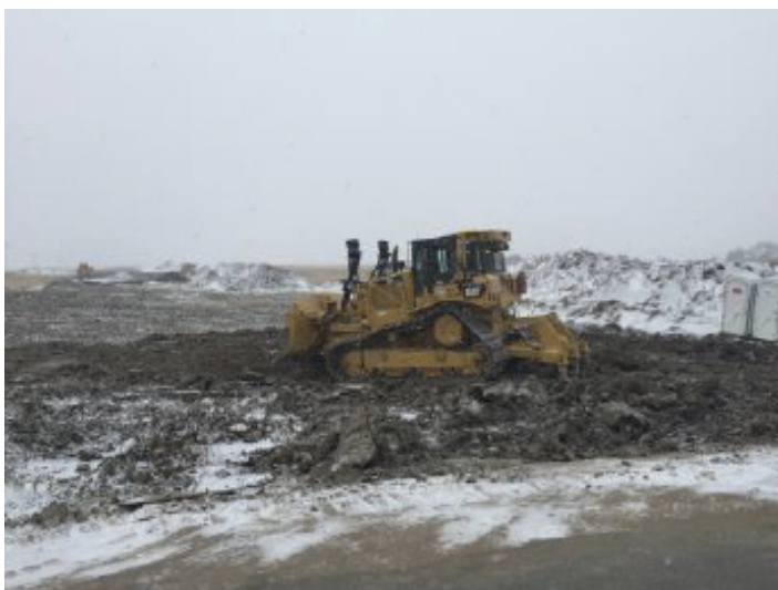
Dozer decompacting sub soil - SF 34 – Nov 9, 2018
