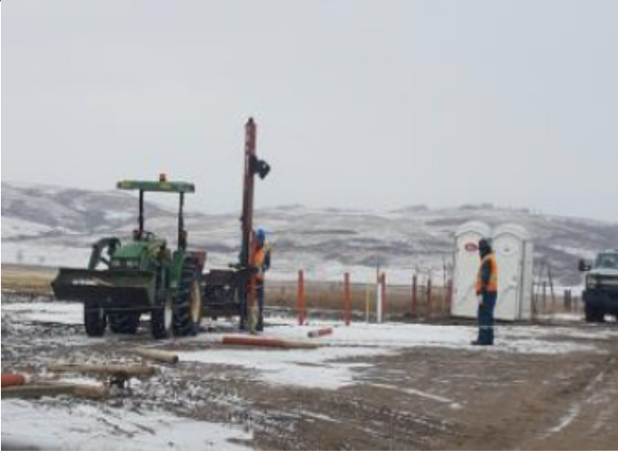
Fencing crew putting up posts – SF 27 – Nov 6, 2018
