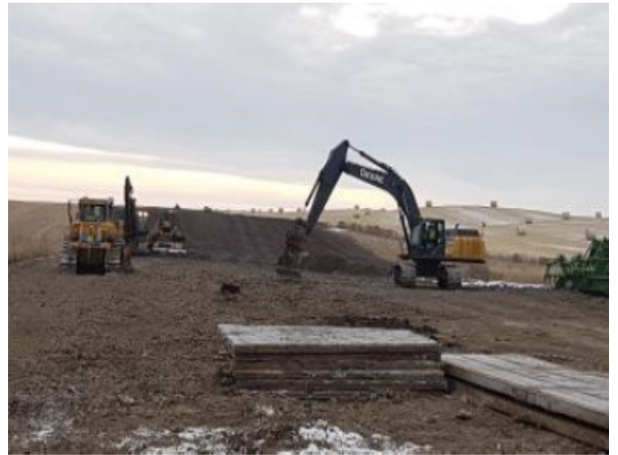
Excavator and dozer breaking up subsoil – SF 52 – Nov 9, 2018
