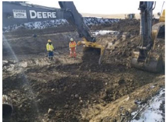
Pipe shading completed– SF 22 – Nov 10, 2018
