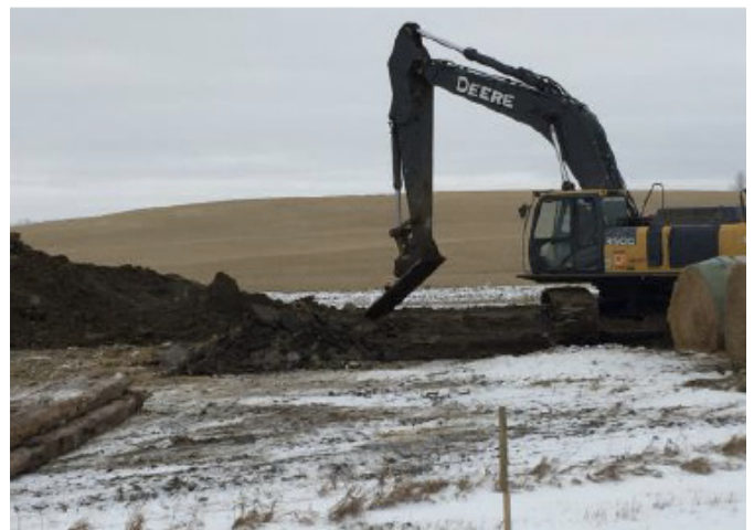
Ovality dig exposed pipe– SF 19 – Nov 8, 2018
