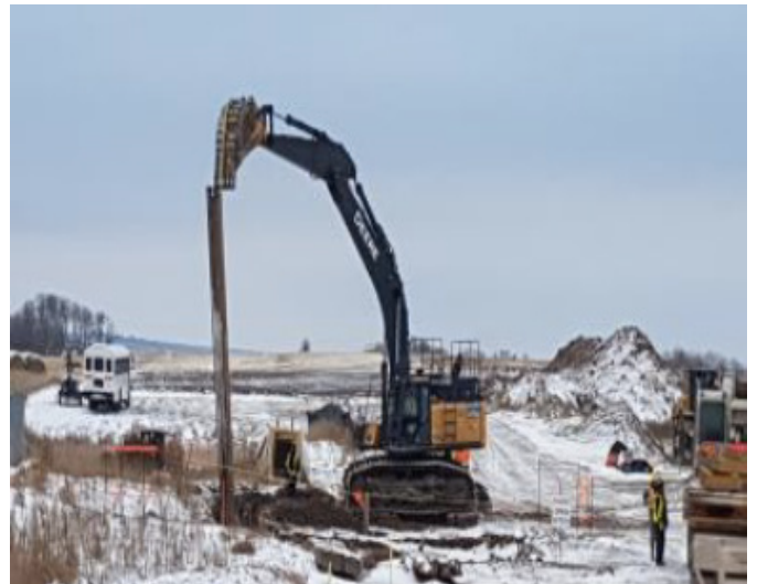
Excavator installing sheet piling – SF 61 – Nov 10, 2018
