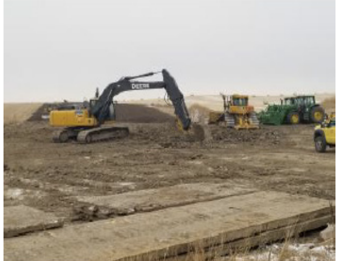
Dozer ripping subsoil – SF 52 – Nov 9, 2018
