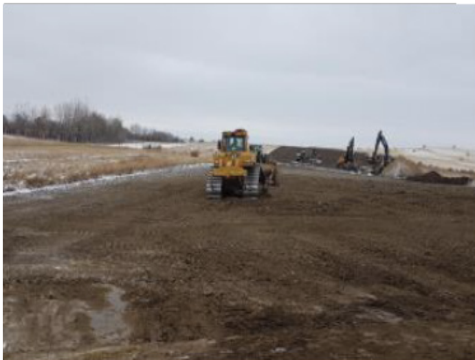
Dozer decompacting subsoil - SF 52 – Nov 10, 2018
