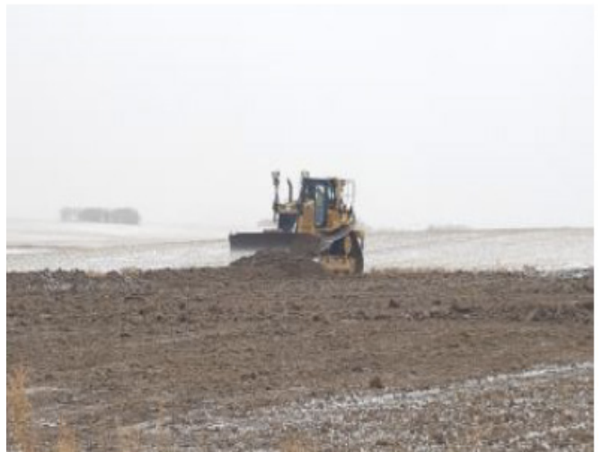
Dozer spreading topsoil – SF 76 – Nov 7, 2018
