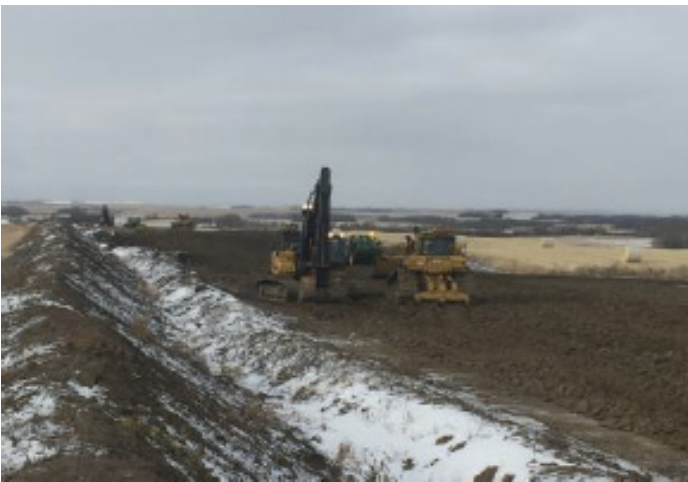
Decompacting sub soil – SF 52– Nov 6, 2018
