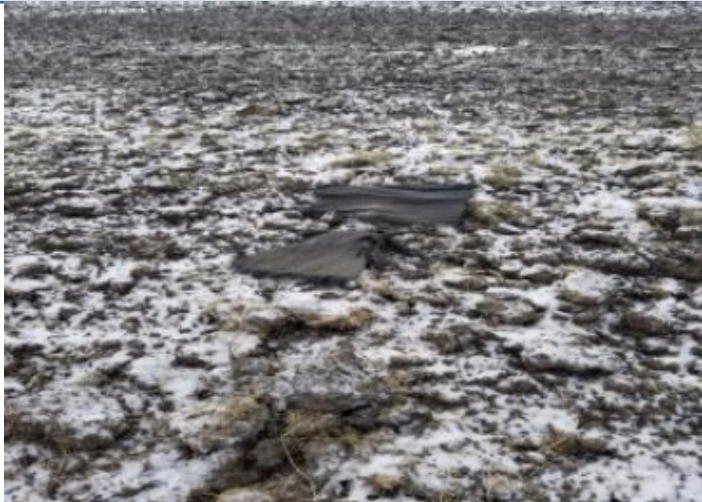
Geotec scattered through ROW – SF 51 – Nov 8, 2018
