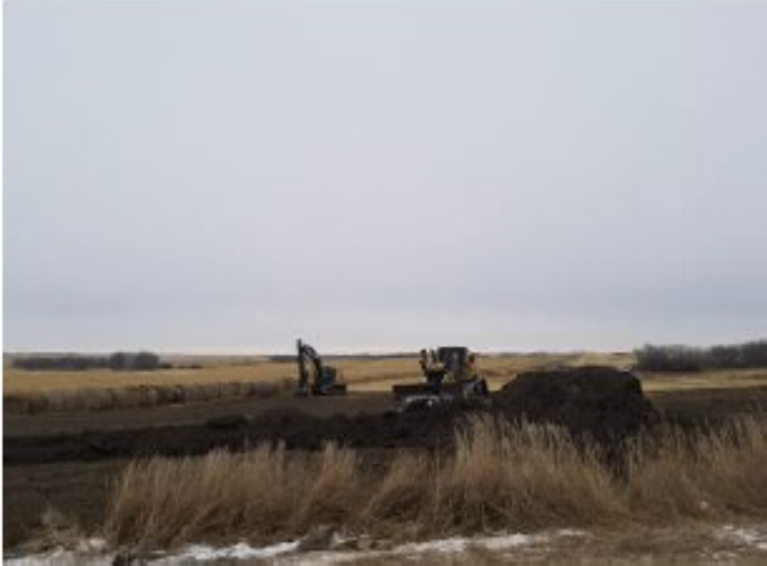
Last of topsoil placement - SF 51 – Nov 9, 2018
