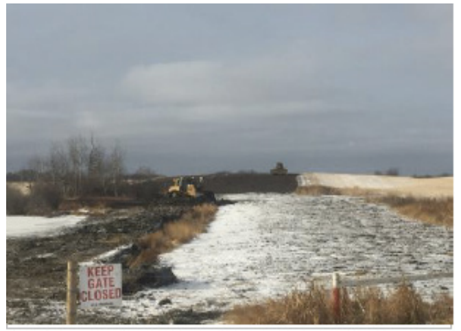
Dozer spreading topsoil – SF 51 – Nov 6, 2018
