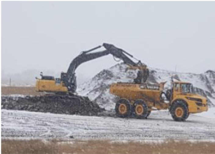
Excavator loading soil on rock truck - SF 34 – Nov 9, 2018
