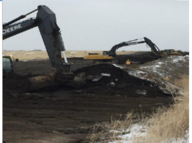
Excavators pulling topsoil – SF 52 – Nov 7, 2018
