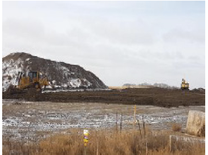
Dozer and excavator spreading topsoil– SF 75 – Nov 5, 2018
