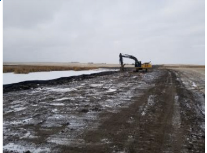
Silt fence installation through wetland – SF 51 – Nov 8, 2018
