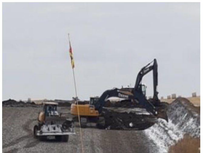
Excavator pulling transition and topsoil– SF 52 – Nov 8, 2018
